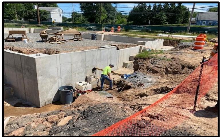
Tomco Pressure Tesing Waterline
