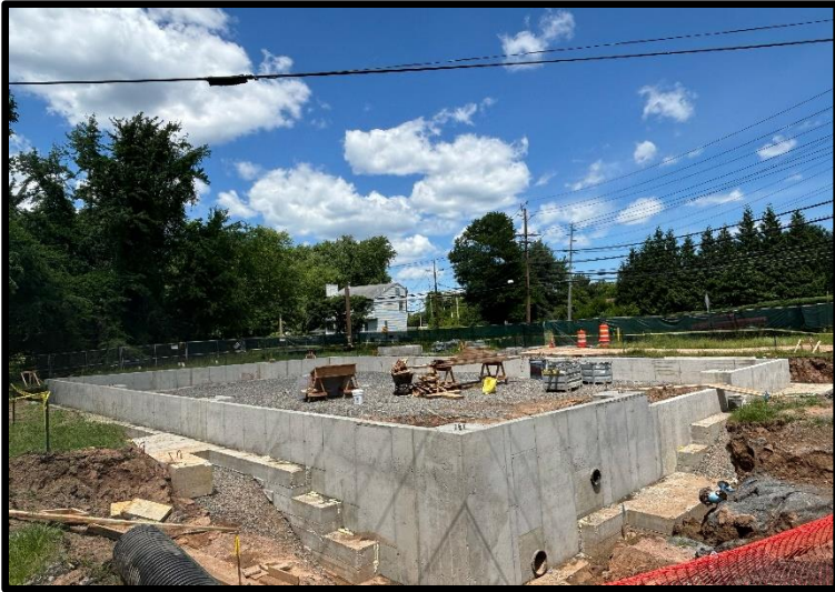
Building Foundation Wall Southwest Corner
