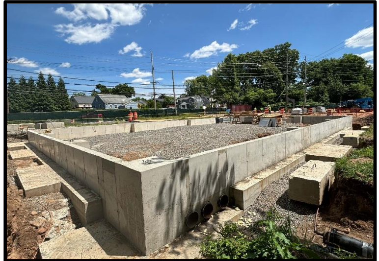
Building Foundation Wall Northwest Corner
