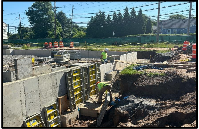
JR Prisco Removing Forms from Foundation Westside Wall
