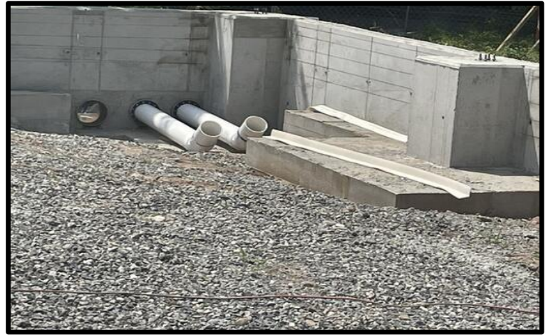
Waterline Piping Under the Sub Slab
