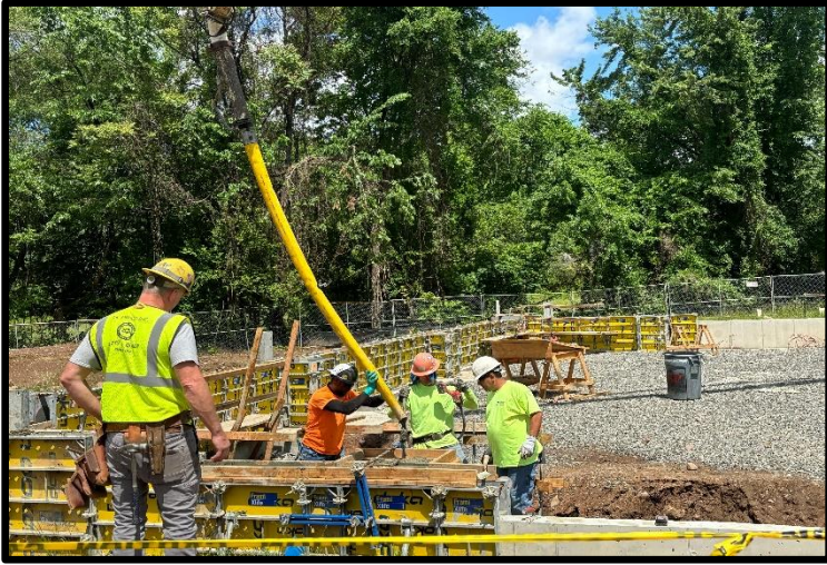
JR Prisco Pouring Concrete Foundation Wall Westside
