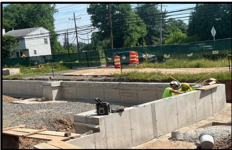
JR Prisco Installing Water Stop Gaps
