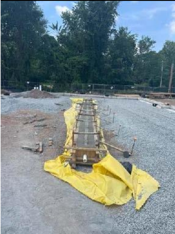
JR Prisco Poured Concrete into Trench Drain Form
