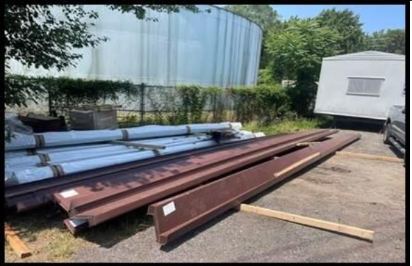
PEMB Structural Material Stored On-Site
