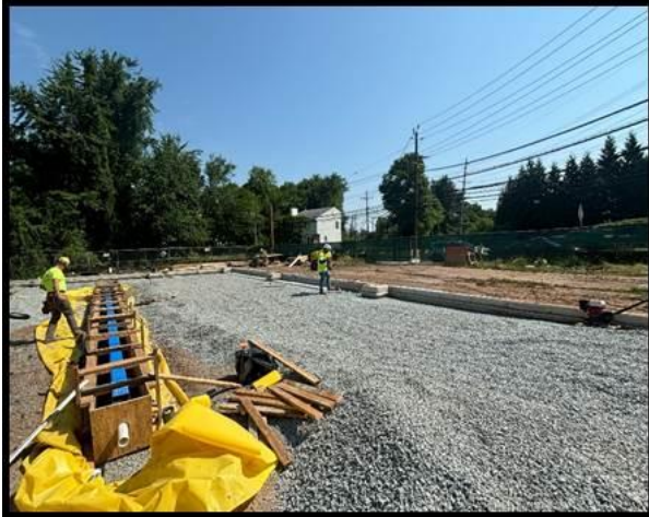
JR Prisco Installing Trench Drain Concrete Form and Piping
