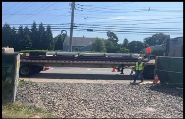
PEMB Structural Material Delivery
