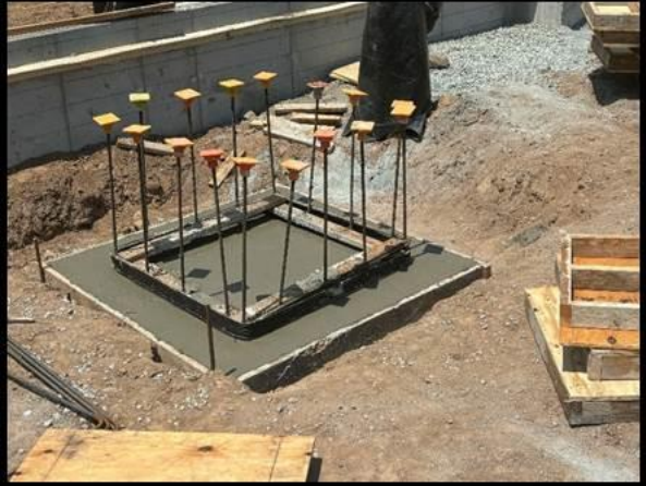
JR Prisco Constructing Sump Concrete Floor Completed Pit Concrete Frame
