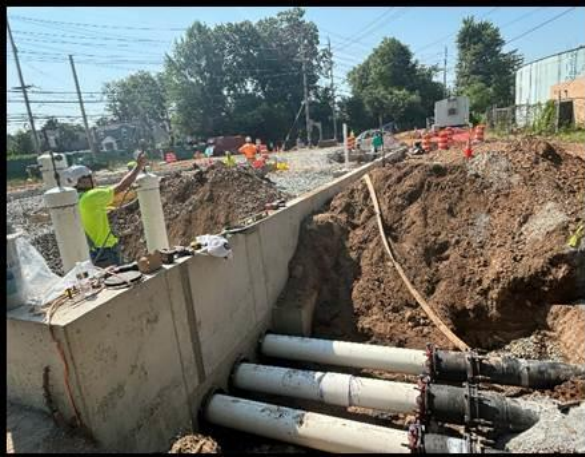
JC Moore Testing Waterlines Entering the Building
