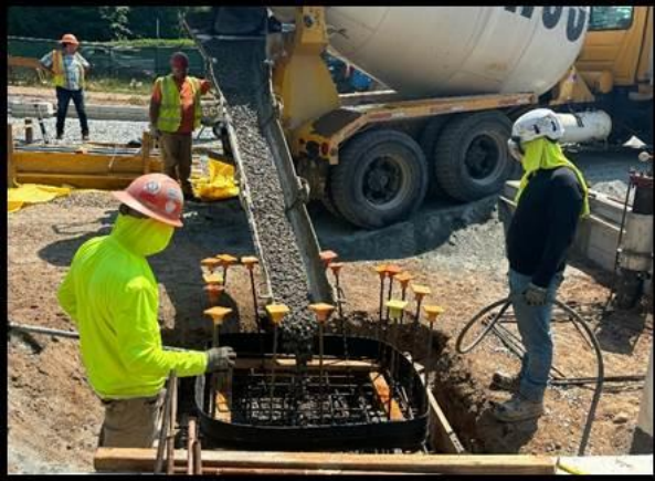
JR Prisco Pouring Concrete for Sump Floor
