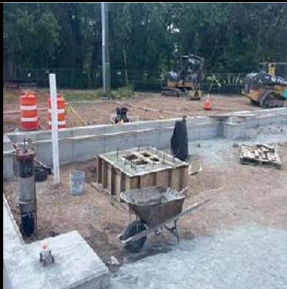
Sump Concrete Box Completed
