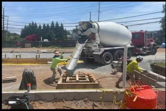
JR Prisco Pouring Concrete into Sump Box Form
