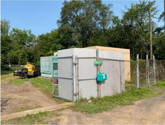
*The foam boards around the fence near the generator that will help reduce noise during operations.*
