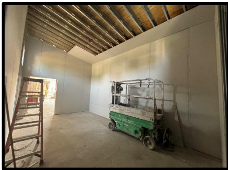
Electrical Room Sheet Rock Buildout
