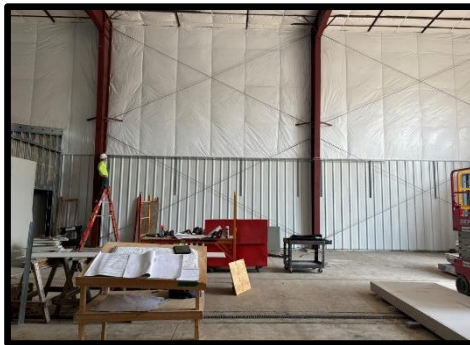
Electrical Service Conduit Installation
