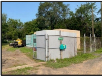
Foam boards to reduce noise from generator.
