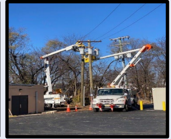
PSEG Working on Power Lines
