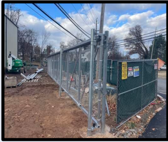
Main Gate Installed
