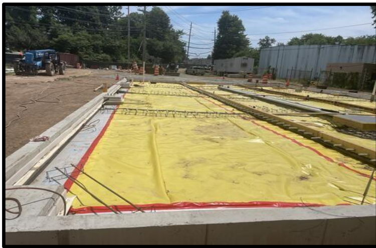
Slab Floor Vapor Barrier Concrete Forms Eastside
