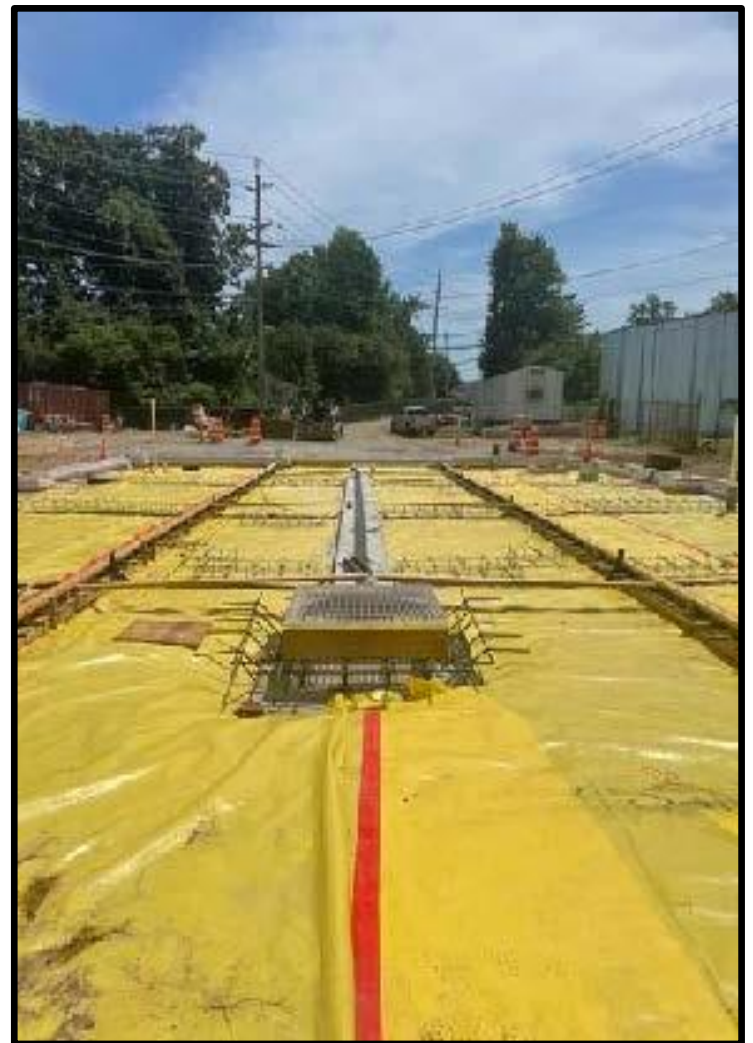
View of Trench Drain, Slip Dowel Concrete Forms, Vapor Barrier Northside
