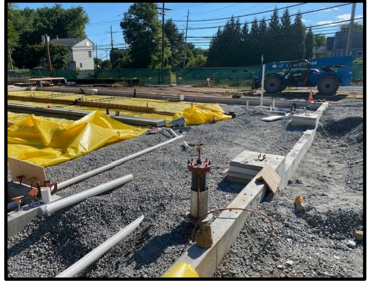
J Moore Installing Piping for trench drain Discharge to Sump
