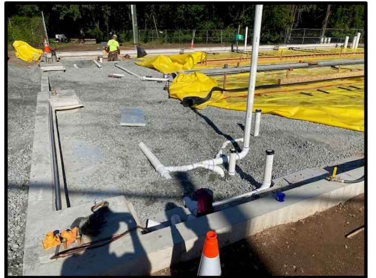
JR Moore Installing Building Bathroom Plumbing/Piping
