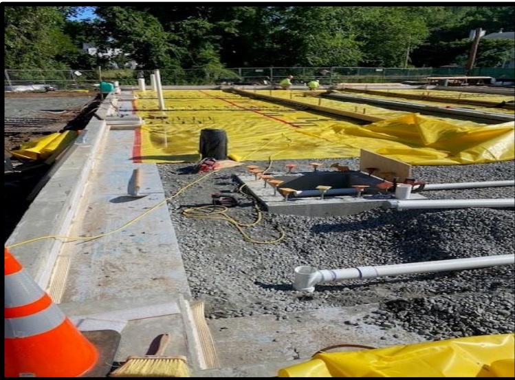
J Moore Installing Discharge Reducer Bag Filter
