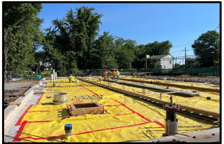
Slab Barrier Southside Sump Sanitary Waterline
