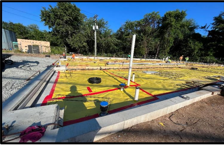
Slab Floor Vapor Barrier Southside Bathroom Location
