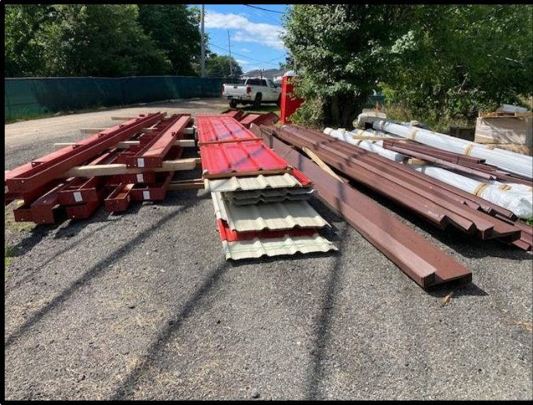
PEMB Structural Material Stored On-Site
