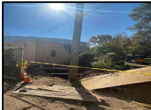
New Power Pole Installed for the FL Pump House
