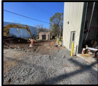
Soil Removal to Reshape Roadway
