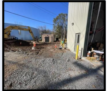
Filling in with Crushed Stone
