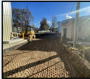
Soil Compacted to Level Driveway
