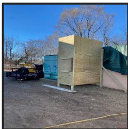
Wood Box constructed to reduce noise from generator.
