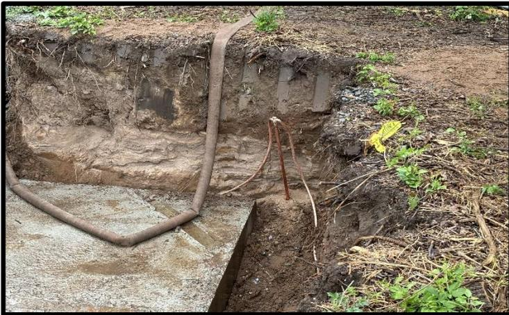
*Installing Grounding Rods Treatment Building*
