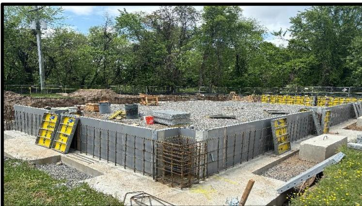
*Finished East Side of Foundation Wall Forms/Panels*
