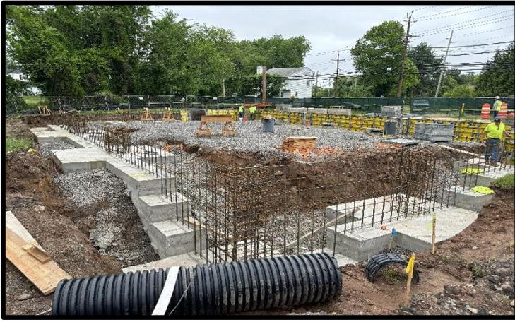
*Finished Foundation Wall Rebar*
