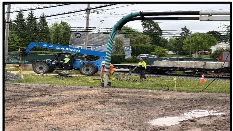
*Soft Digging for Gas Electrical and Water Pipelines*
