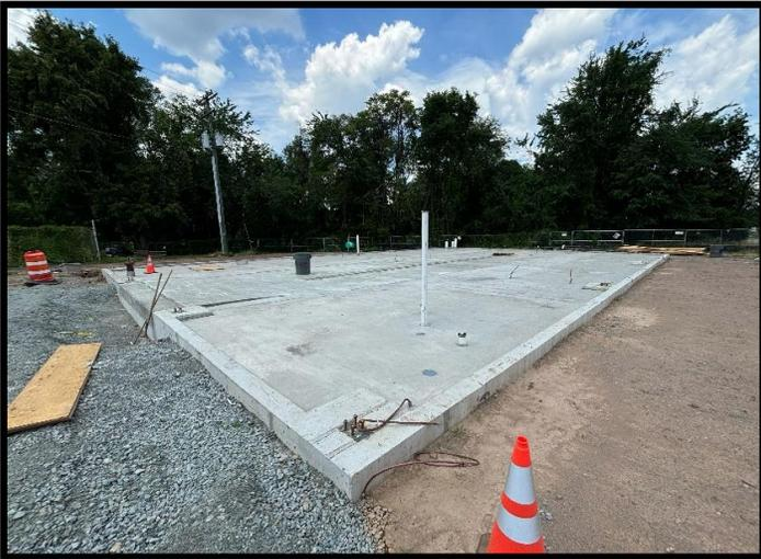
Finished Building Concrete Slab/Floor
