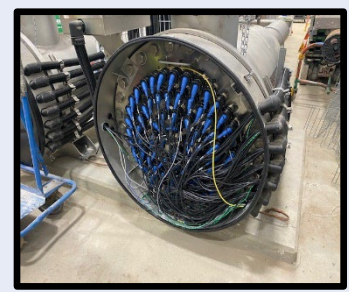
UV/OX Bulb Wiring
