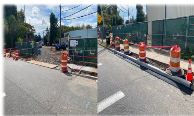
New Curb Installation for Site Entrance
