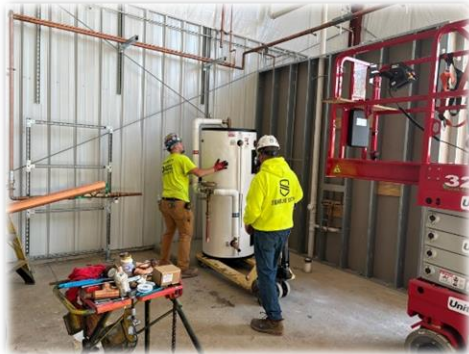
Water Heater Installation
