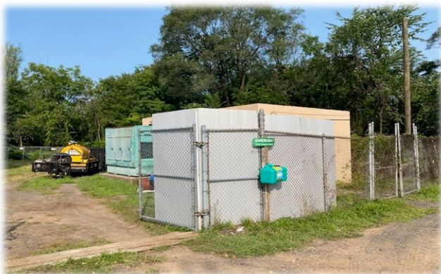
Foam Boards Around Fence to Reduce Noise from Generator Operations
