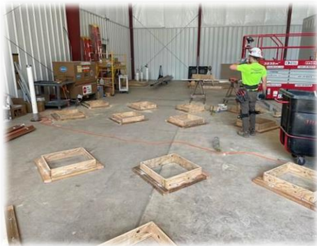
Indoor Concrete Pad Framing
