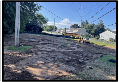
Regrading of Soil Along Westmoreland Ave.
