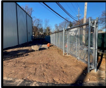
Permanent Fencing 11st Street Side
