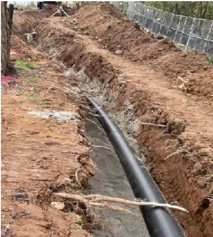
Clean Water Pipe Installed Underground
