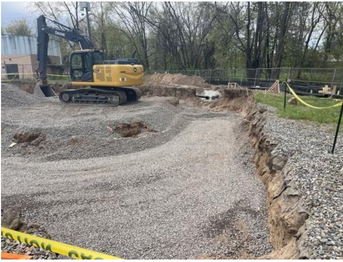
Foundation Base Back filled with Crushed Stone
