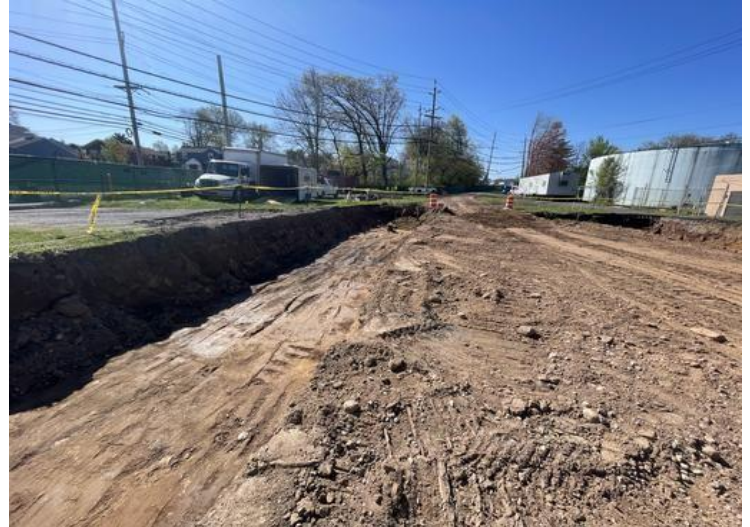
Building Foundation Excavation
