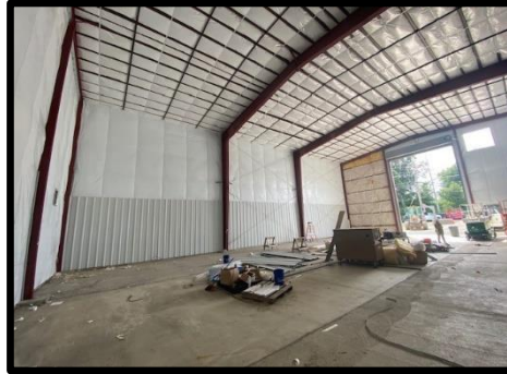
Building East Side Interior Wall Insulation and Paneling
