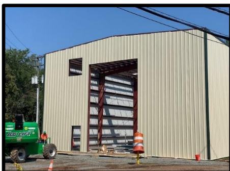
Front Side of the Building
